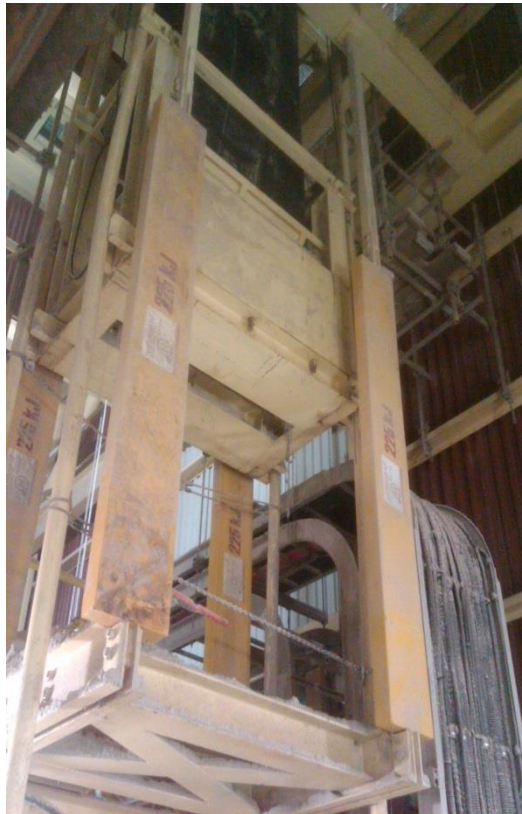
View of Technogrids® and catch frame from underneath installation.
